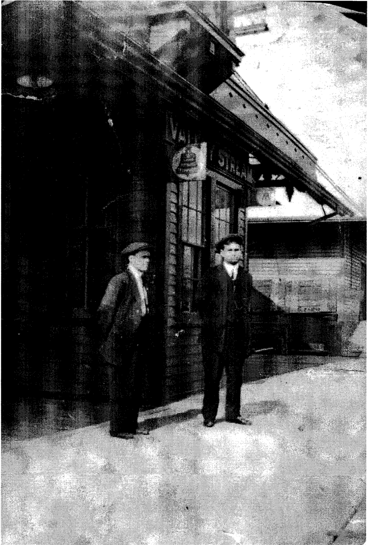
Valley Stream Rail Road Station at Rockaway Avenue
